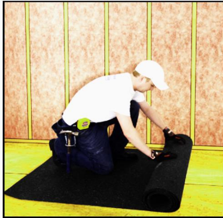
Place the roll of BlastBlock on the floor, then cut to length
